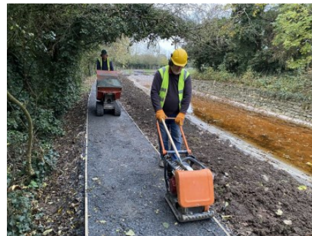
Improvement works in progress close to Crickheath Bridge.
