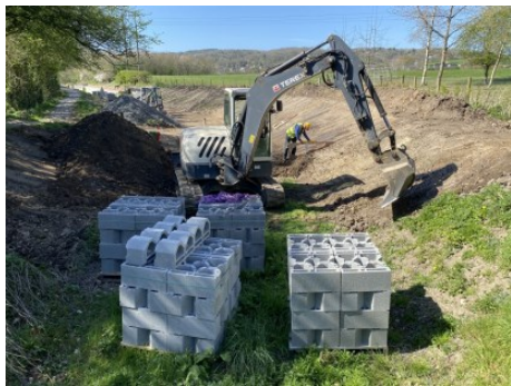
Temporary dam now ready to be removed
