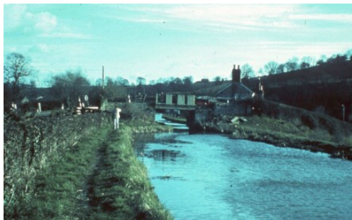
Williams Bridge before demolition in 1980 (photo: Waterways Images)
